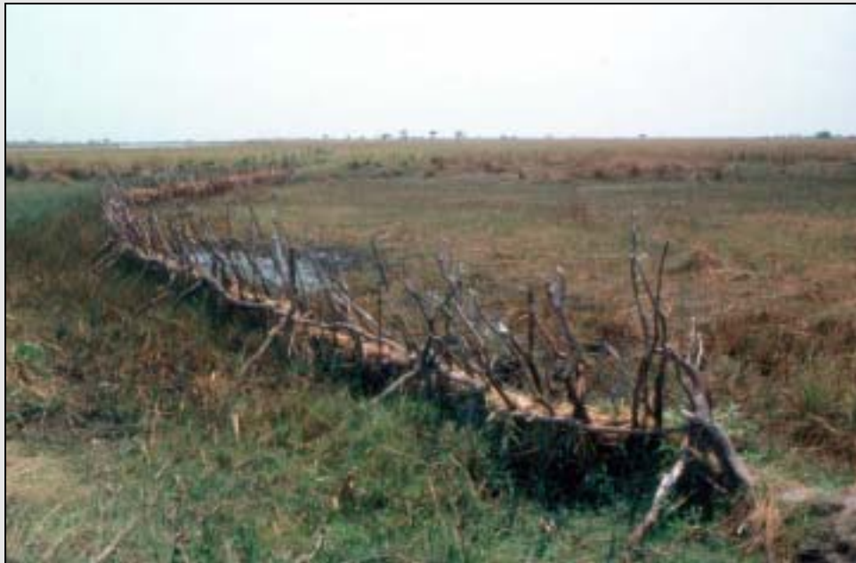
Photo 9: Permanent walilo structure on Zambezi Westbank floodplain, Zambia, during dry season
